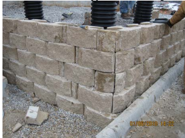
Admin Bldg retaining wall
