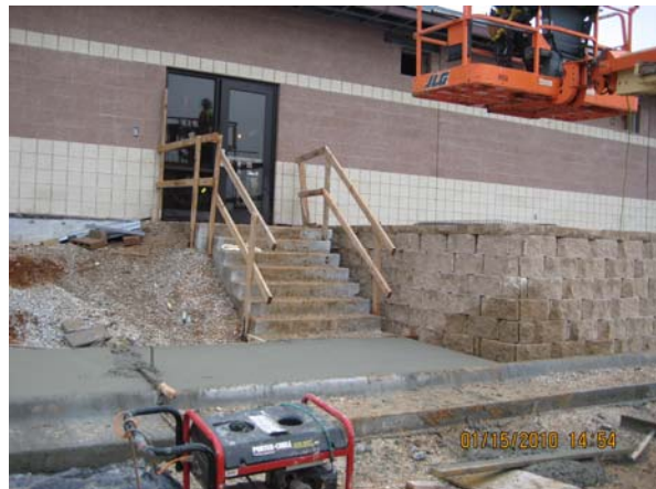
Admin. Bldg. back entrance
