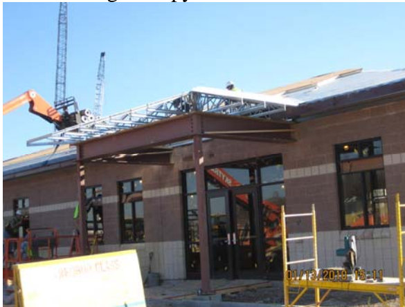
Admin. Bldg. entrance
