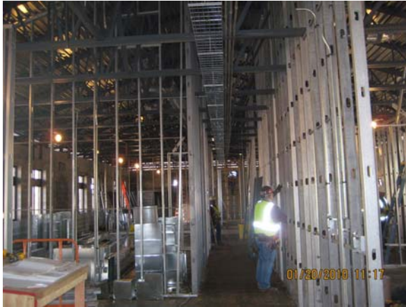
Interior walls at Admin. Bldg.
