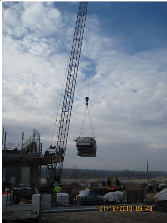
Belt Filter Press hoisted into building
