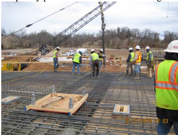
Placing concrete for Process Train 41 north deck
