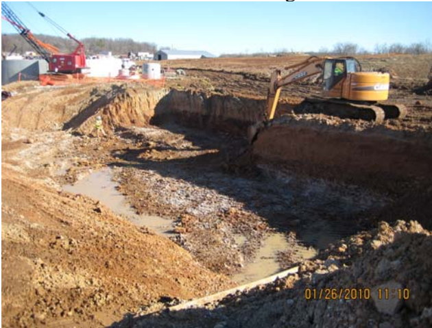
Filter Bldg. excavation
