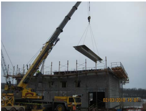
Setting precast roof tees on Sludge Process Bldg.
