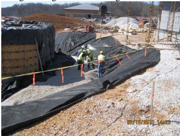
Backfilling Grit Chamber
