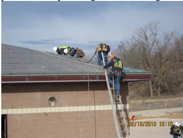
Beginning installation of metal roofing sheets
