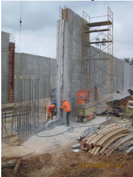
Demolition of Process Train wall 74
