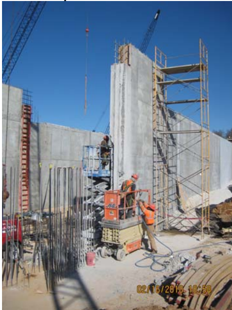
Process Train wall 74 demolition
