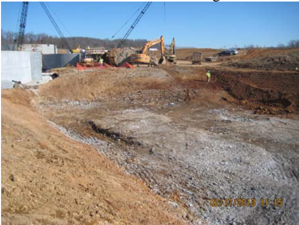
Filter Building excavation
