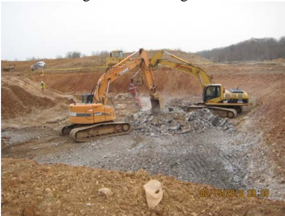
Rock excavation at filter bldg.
