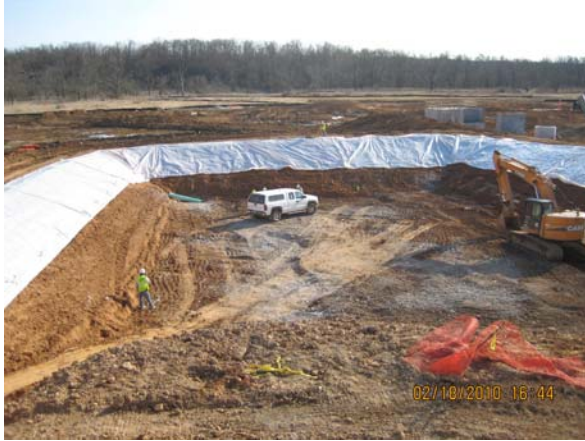
Filter Building excavation
