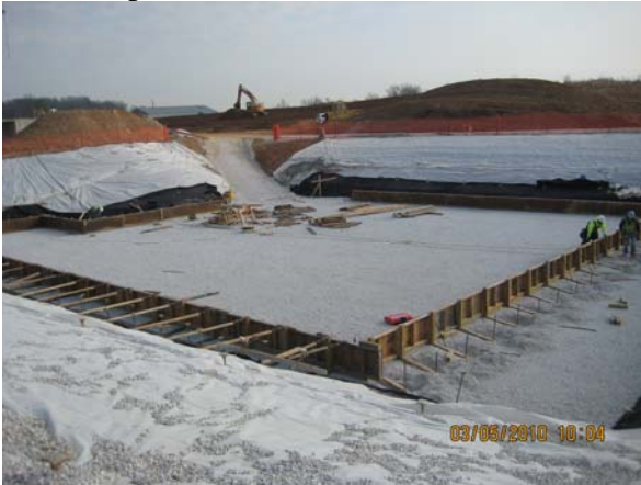
Filter excavation looking Northeast
