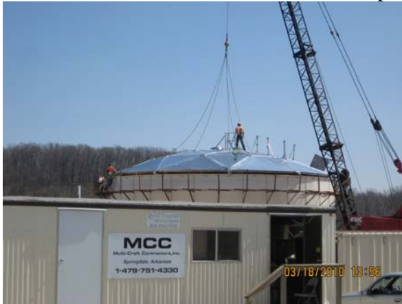
Setting dome on top Supply Water Tank
