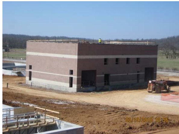
Sludge Process Bldg.
