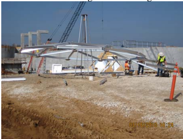
Water Supply Tank dome assembly
