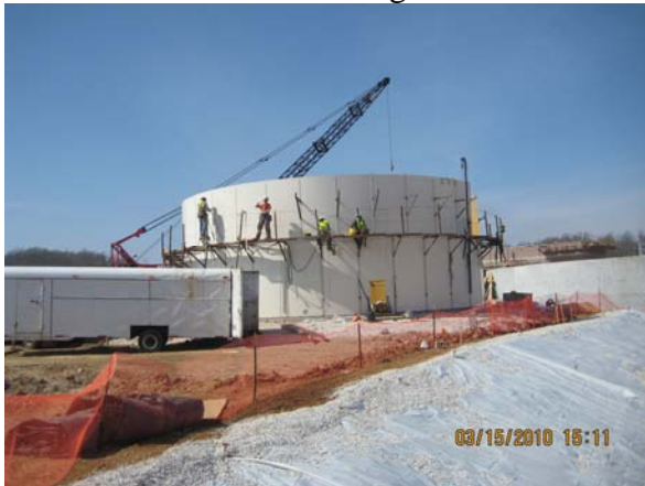
Water Supply Tank erection
