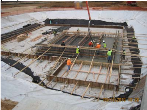
Concrete placement of NW quadrant of filter bldg base slab
