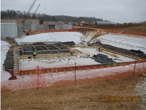
Filter Bldg base slab
