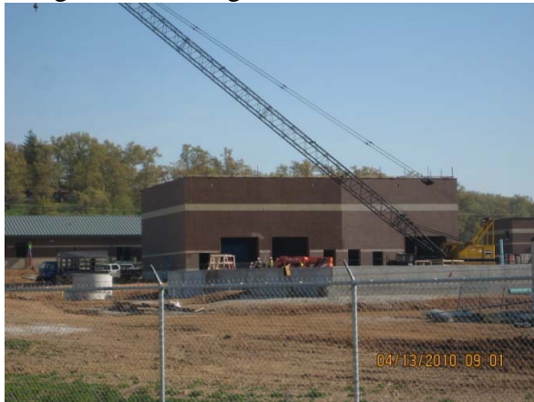
Sludge Process Bldg. exterior block half sealed
