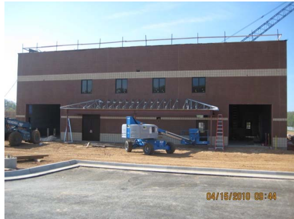
Sludge Process Bldg.
