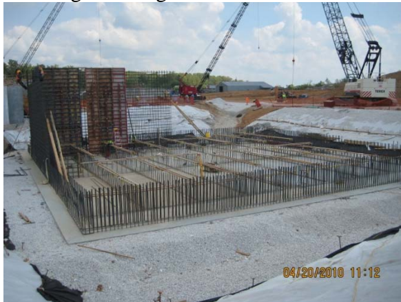
Erecting forms for filter bldg. walls
