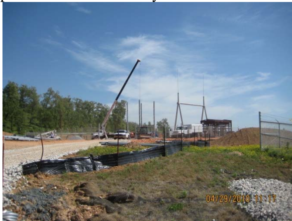
Carroll Electric Substation steel erection
