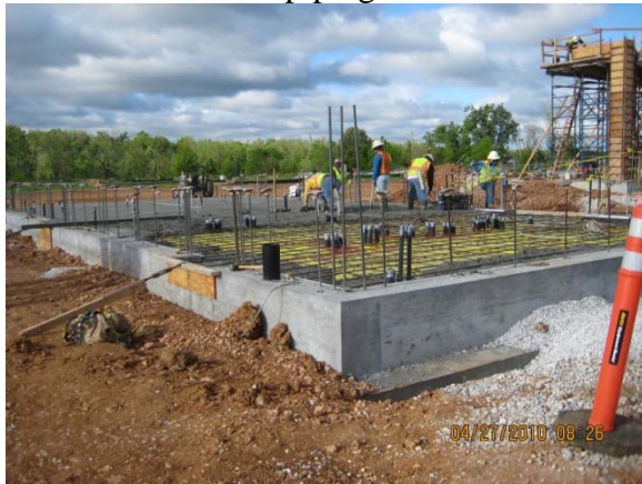
Placing concrete for Control Bldg. #1 floor.
