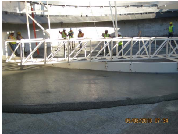
Placing grout for Clarifier 61 floor.
