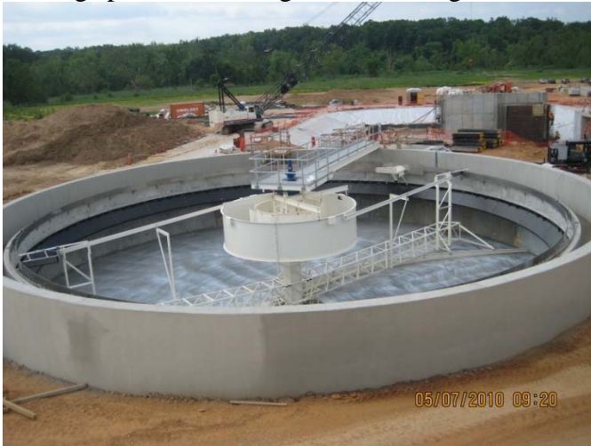
Clarifier 61 with poured floor
