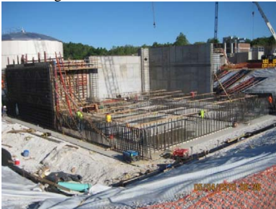
Filter Bldg. looking NW
