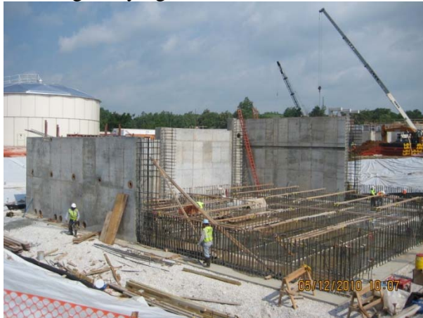
Filter building looking Northwest
