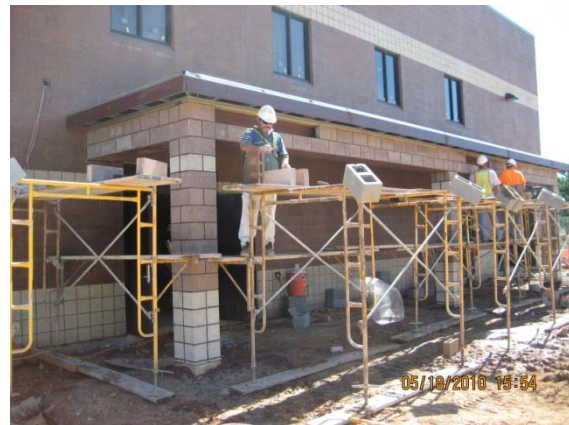
Sludge Process Bldg. canopy masonry
