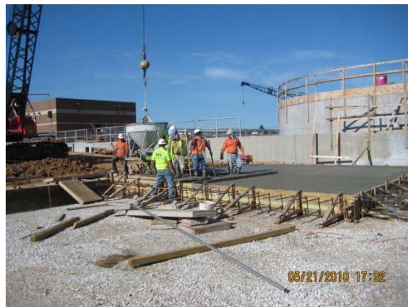
Placing concrete for NE ¼ of NW crane pad
