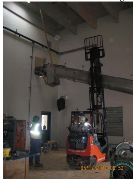
Setting inclined sludge conveyor in Sludge Process Bldg.
