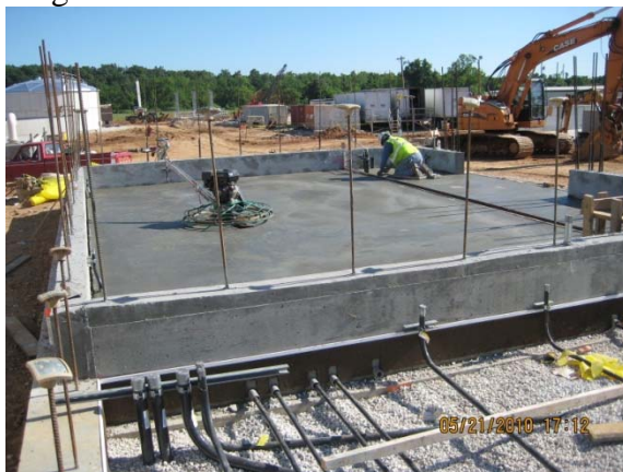
Finishing Control Bldg. #2 south floor slab
