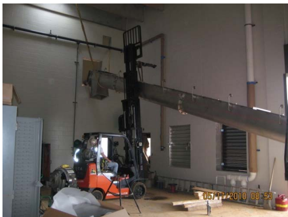
Setting inclined sludge conveyor in Sludge Process Bldg.
