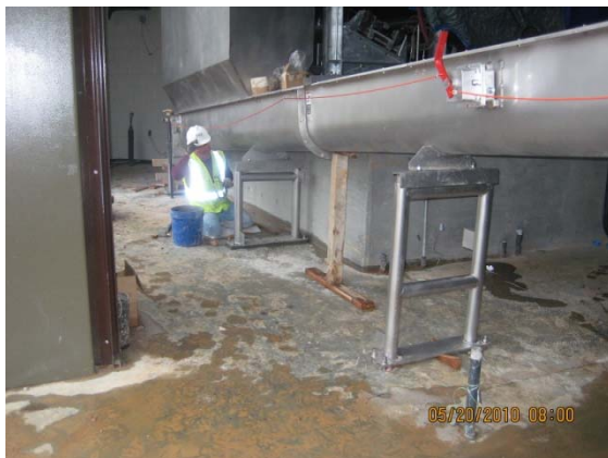
Grouting sludge conveyor supports
