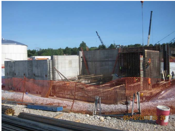
Filter bldg. looking NW
