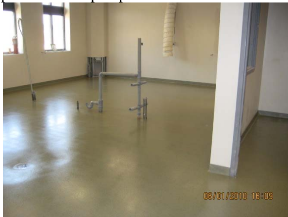
Resinous floor in Admin. Bldg. lab
