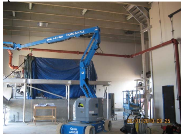
Installing sludge piping in Sludge Process Bldg.
