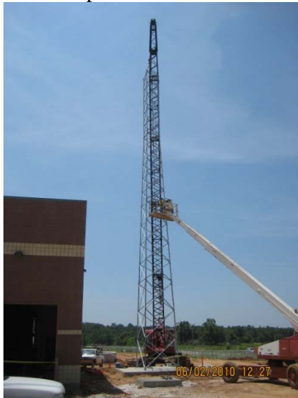
Setting radio tower west of Sludge Process Bldg.
