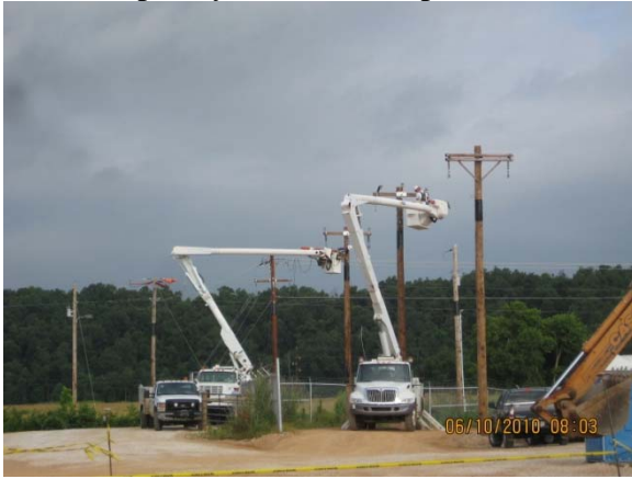
Stringing power lines into treatment plant
