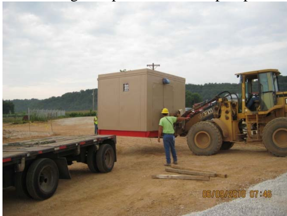
Fire Pump Enclosure being unloaded
