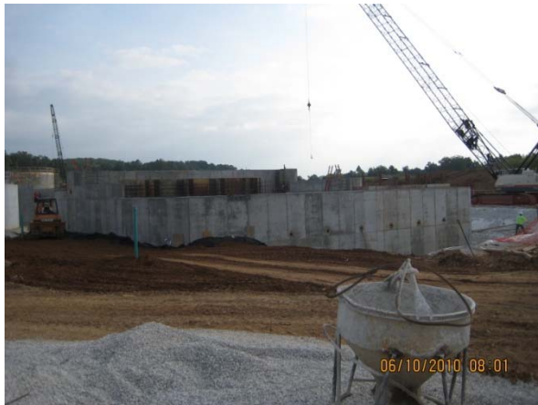
Filter building looking Northeast
