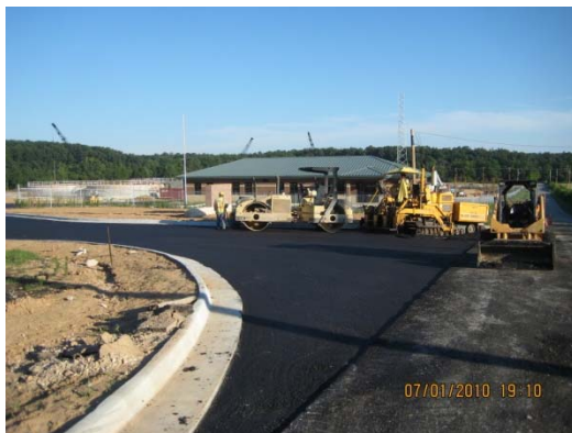
Asphalt paving Main Entrance Road and Plant Road #1
