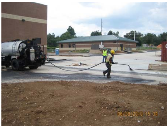
Photo 1: Prime Coat Application
