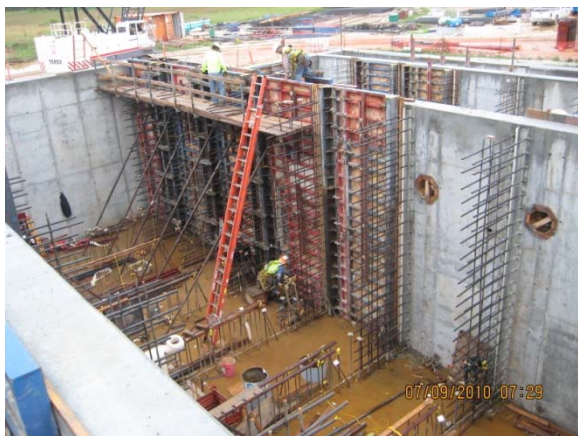
Southeast corner of Filter Bldg.
