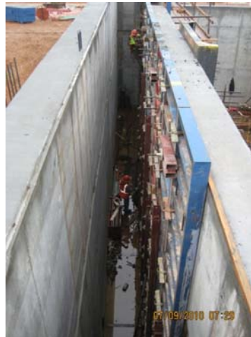
Northeast corner of Filter Bldg.
