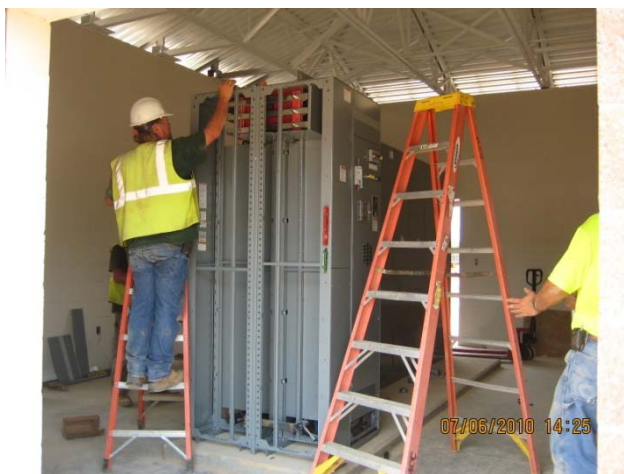
Photo 1: Installing MCC at Control Building No. 1.
