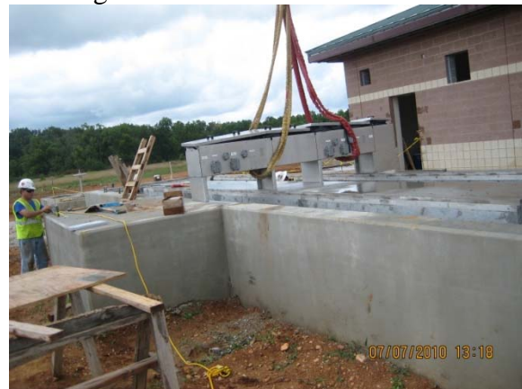
UV Equipment being set in place
