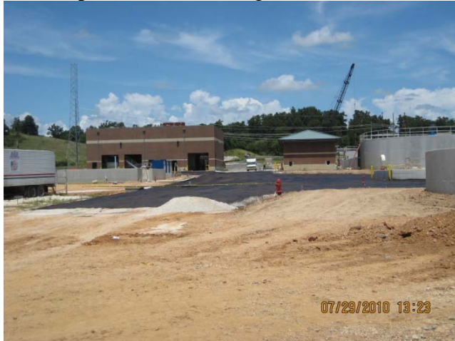
Sludge Process Bldg. & Control Bldg. #2
