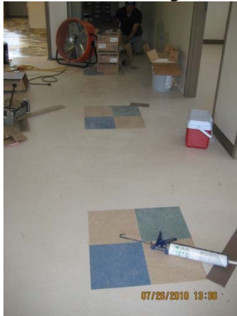
Admin Bldg floor tile
