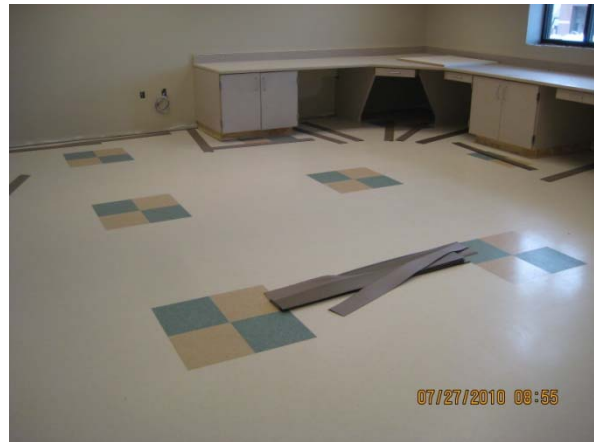
Admin. Bldg. Control room
