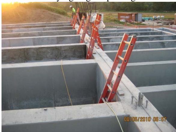
Filter Bldg. interior walls
