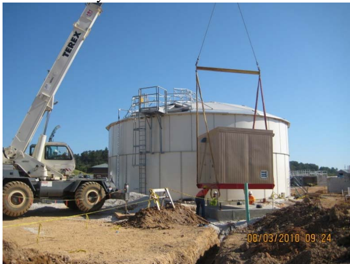
Setting Water Tank pump station enclosure
