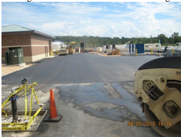
Paving Plant Road #1
