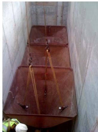
Cone sections set in filter bldg.
