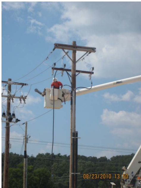
Terminating cables at Carroll Electric power pole
