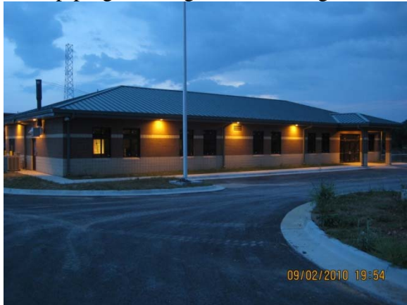
Exterior lighting at Admin. Bldg.
