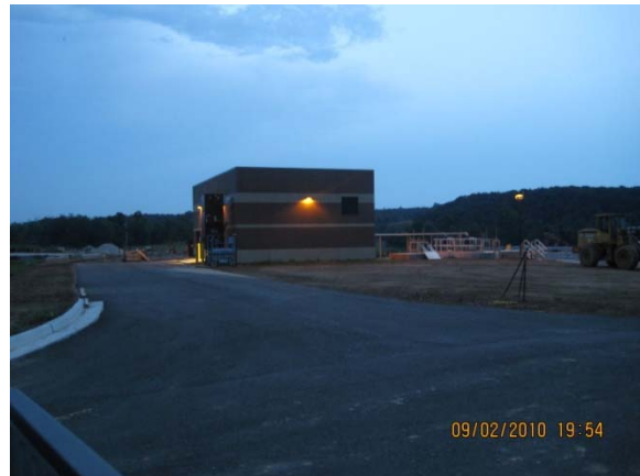
Exterior lights at Screen Bldg.
