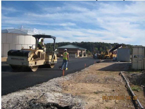
Paving Plant road #1.
