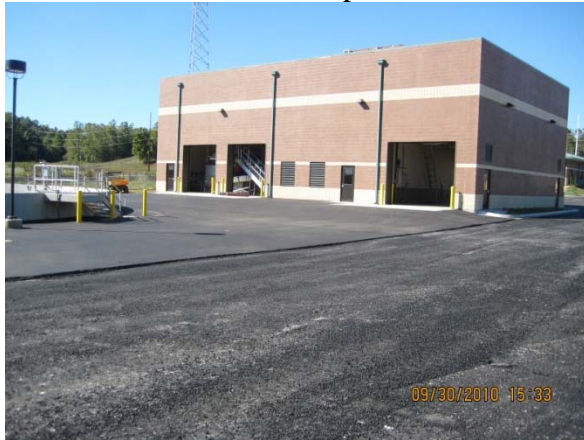
Asphalt paving on south side of Sludge Process Bldg.
