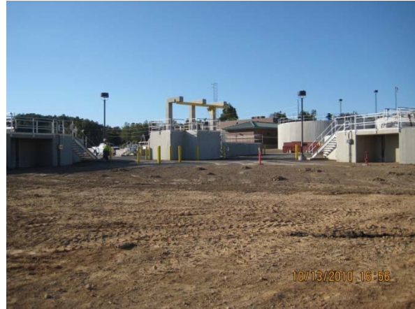
Splitter and clarifiers
