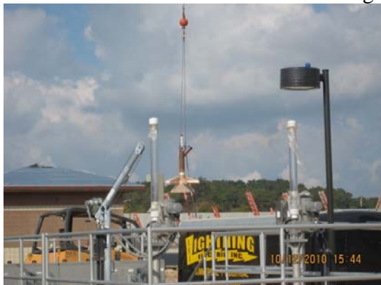
Lowering distributor piping into filter cell
