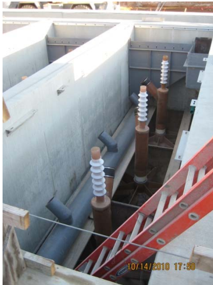
Distributors in filter cells
