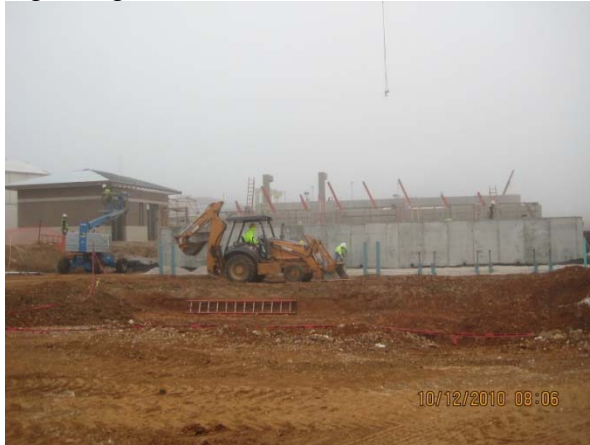
Control Bldg. #3 & Filter Bldg.
